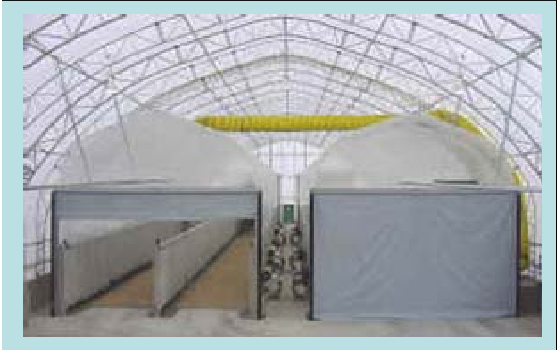
Figure 1.2.2.3: A fully enclosed 10,000 tonnes per year composting facility. (By the permission of Transform Compost Systems.)
