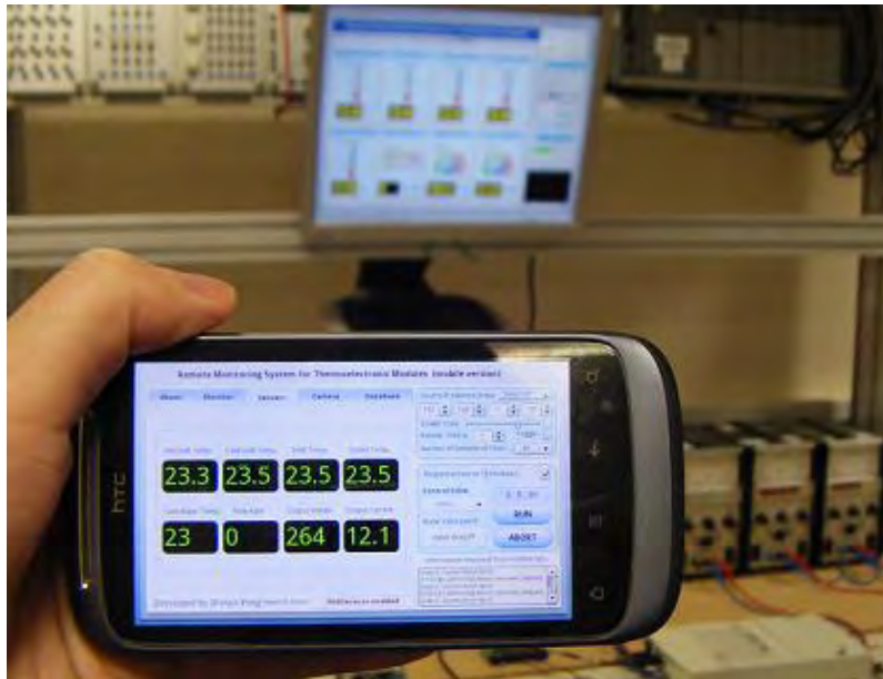
Figure 6.12 Remote acquisition of working condition data from the secondary panel of the server using HTC mobile phone
