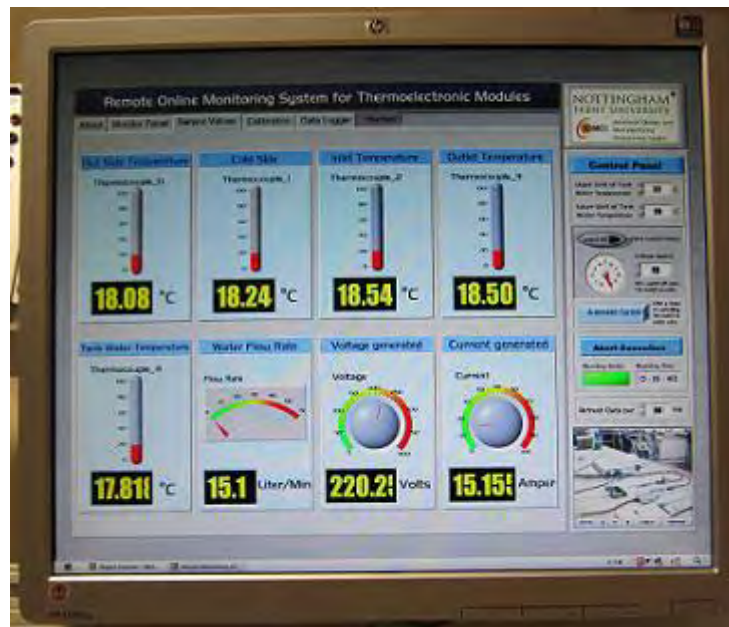
Figure 6.4 Real-time display of working conditions data in the secondary monitoring panels
