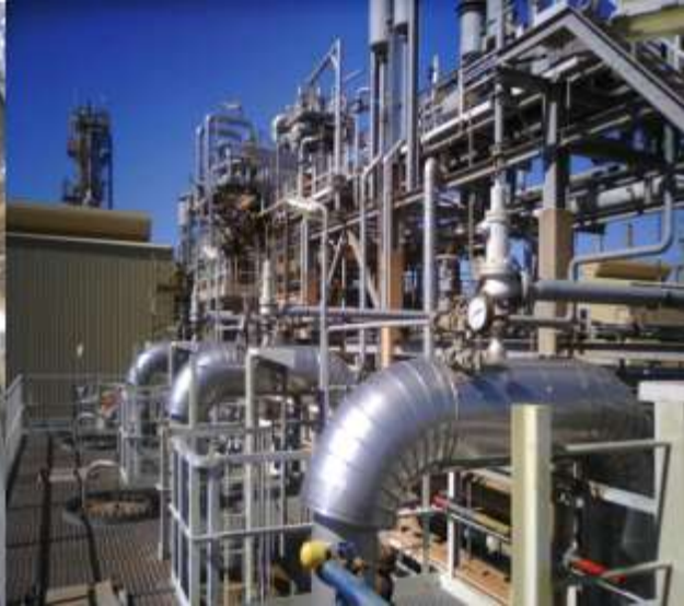
Figure 5:12- Vent lines on dryers
