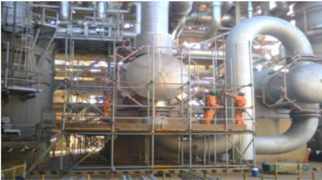
Figure 5:13- Scaffold to exchanger
