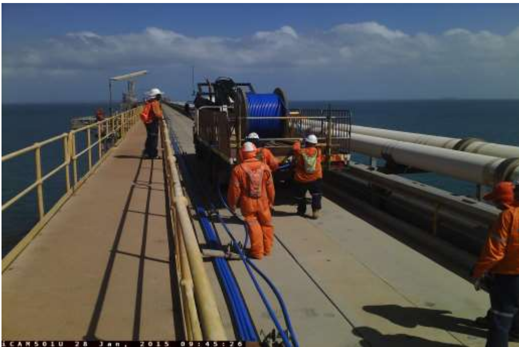
Figure 5:30 - Wagon assisted cable laying
