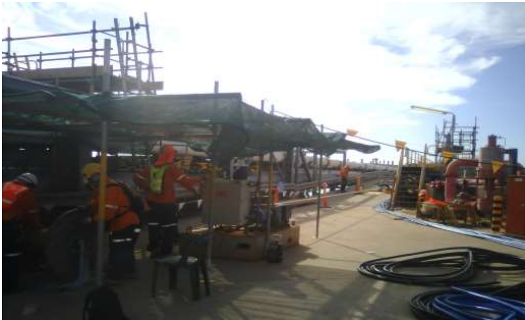
Figure 5:29- Cable pulling using winch
