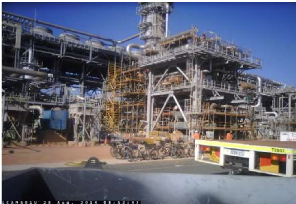
Figure 5:14 completed scaffold access
