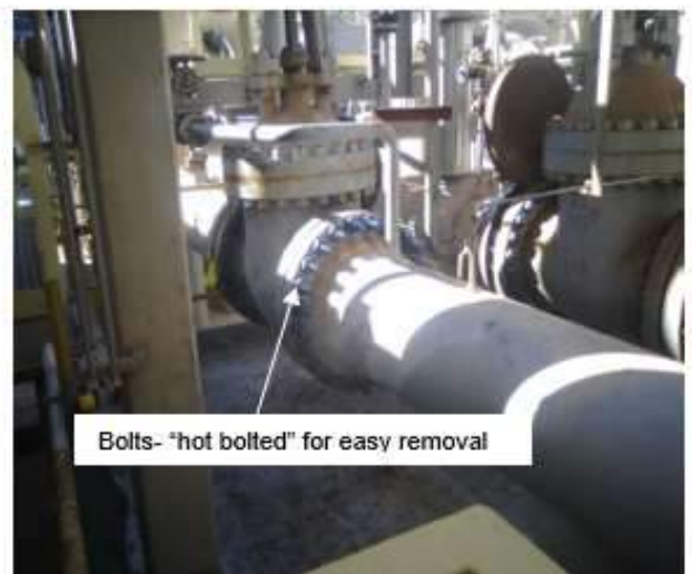
Figure 5:8 - valves "hot-bolted" prior to removal
