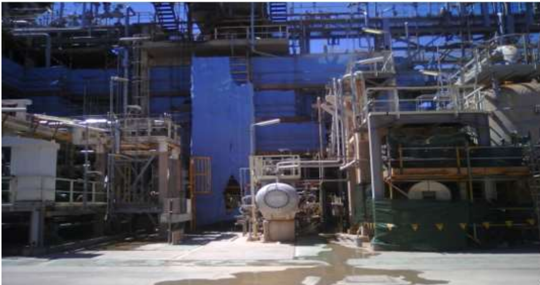
Figure 5:2 -Scaffold for STIPS inspection
