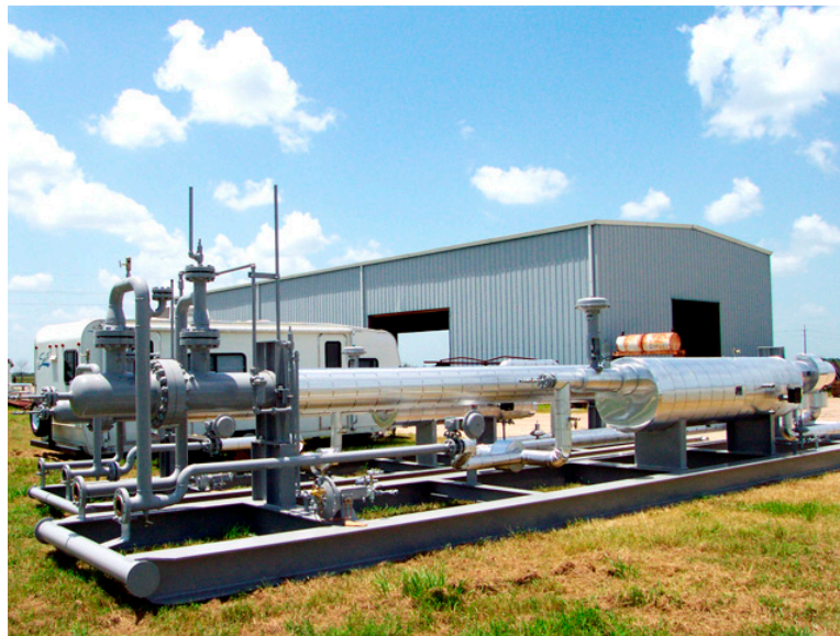
Figure 3. Typical Joule-Thompson low temperature separation (JT-LTS) facility installed in the Yokiri Forcados Integrated Power (FYIP) North Bank Flow Station, Ogulagha Island, Niger Delta. Source: [52].
