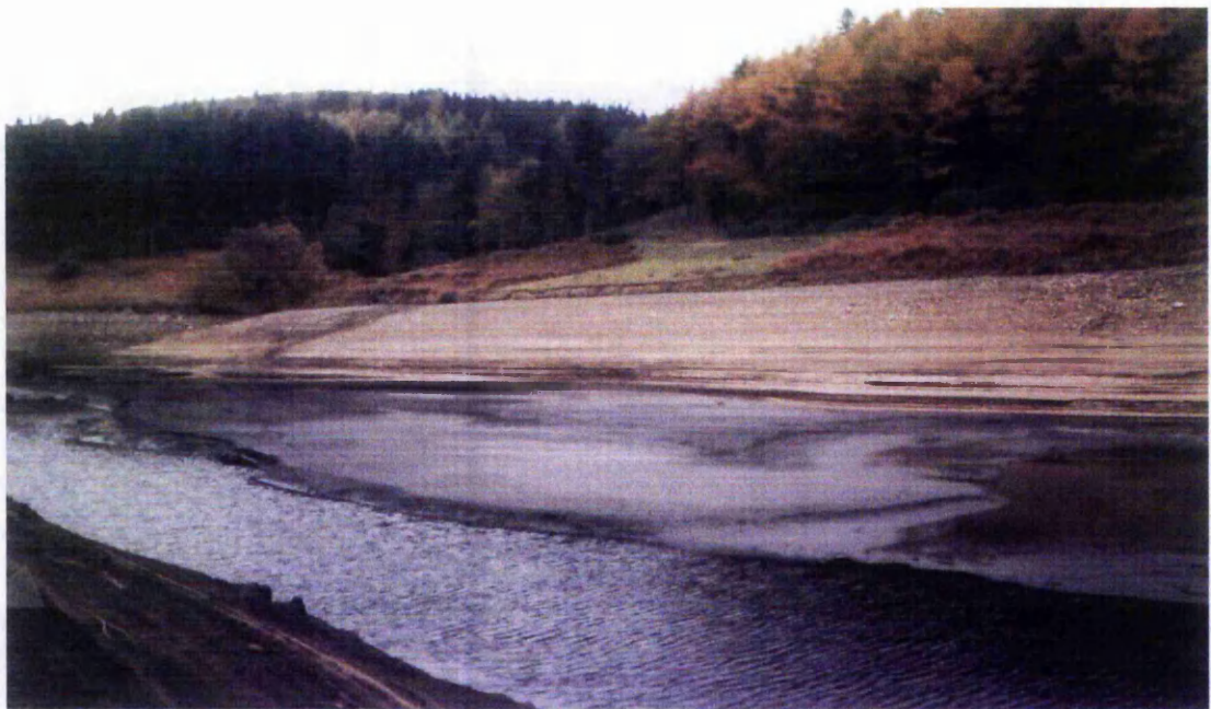
Figure 1.1 Sedimentation at Howden Reservoir - stage nine metres below top water level (Lees, 2003 pers. comm.)
