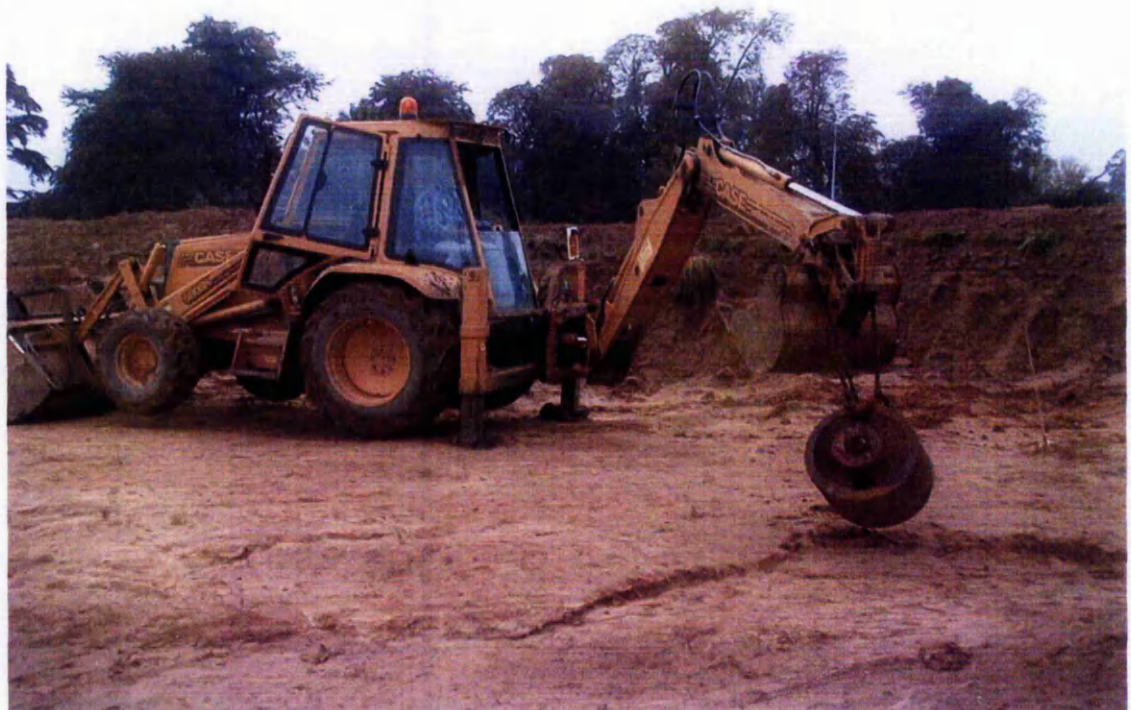
Plate 4.2. Photograph of the investigation site being compacted
