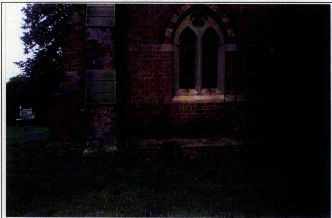
Figure 4.6 - Hoveringham Church. Close up of corner suffering settlement.
