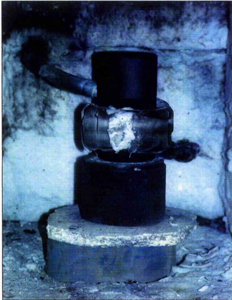
Figure 6.13: Induction coil covered with thermal insulating tape.
