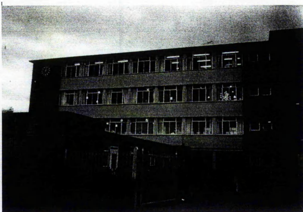
Plate 5.9: School building exterior view
