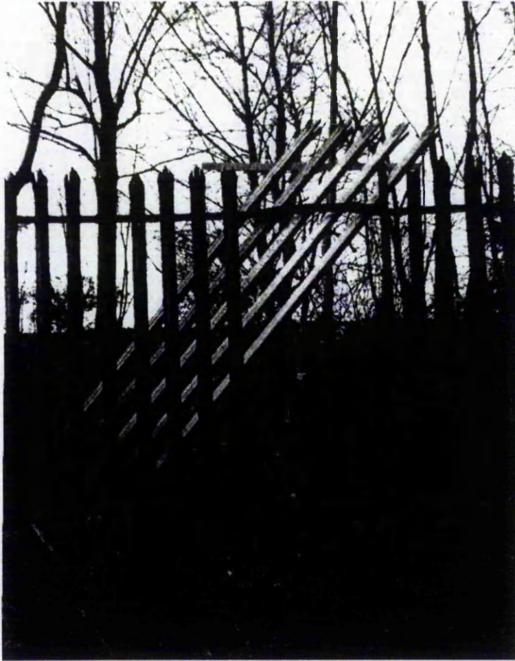
Plate 5.2 Park/towpath security fencing breached by nocturnal activities of cruisers
