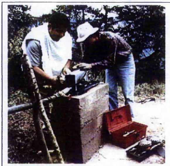
Figure 2-4 Installation of an FTDA Pelton turbine.
