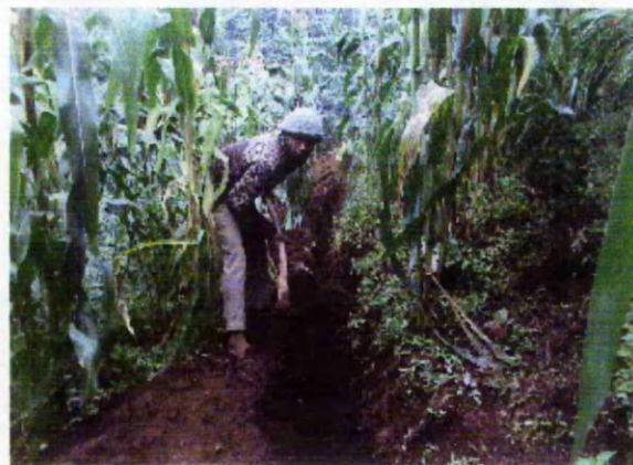
Digging the penstock trench
