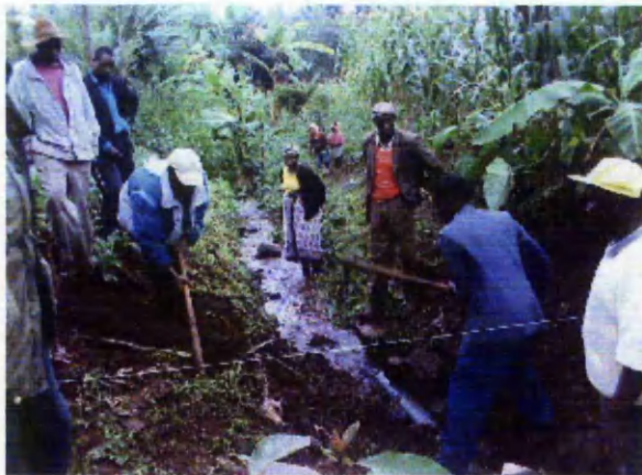
Preparing foundations for the weir
