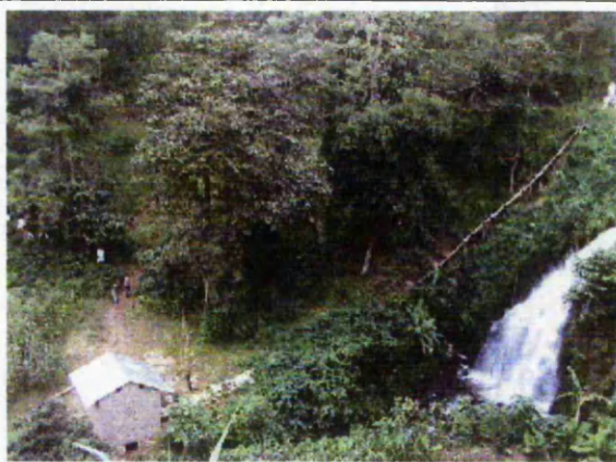
This scheme was installed in 10 days at a cost of $2,600 (excluding distribution and house wiring).
