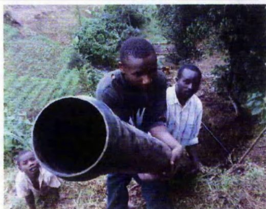
Sockets enable the 6m pipe lengths to be fitted together. An 'O' ring fits in the socket recess and provides a pressure tight seal.
