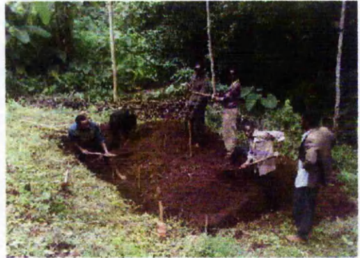
Digging out the footing for the walls.
