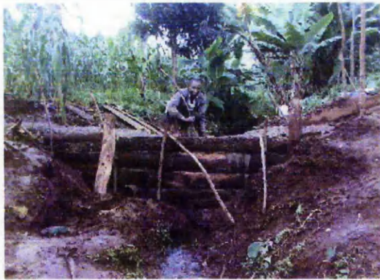
Shuttering in place during application of cement layer to seal the weir
