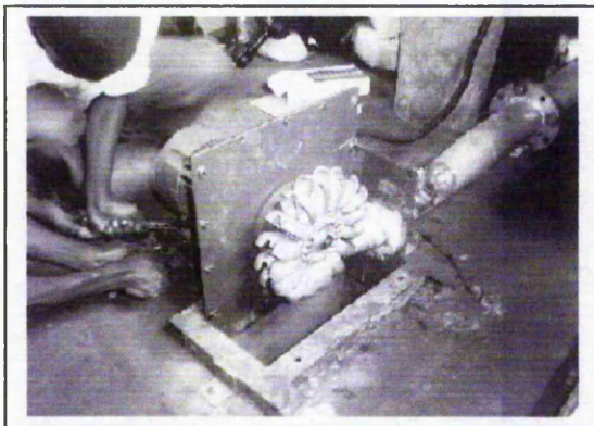
Figure 4 1.1 kW Pelton Turbine, Kathamba
