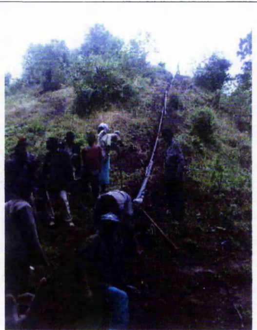
Laying the pipe from the intake to the turbine house.
