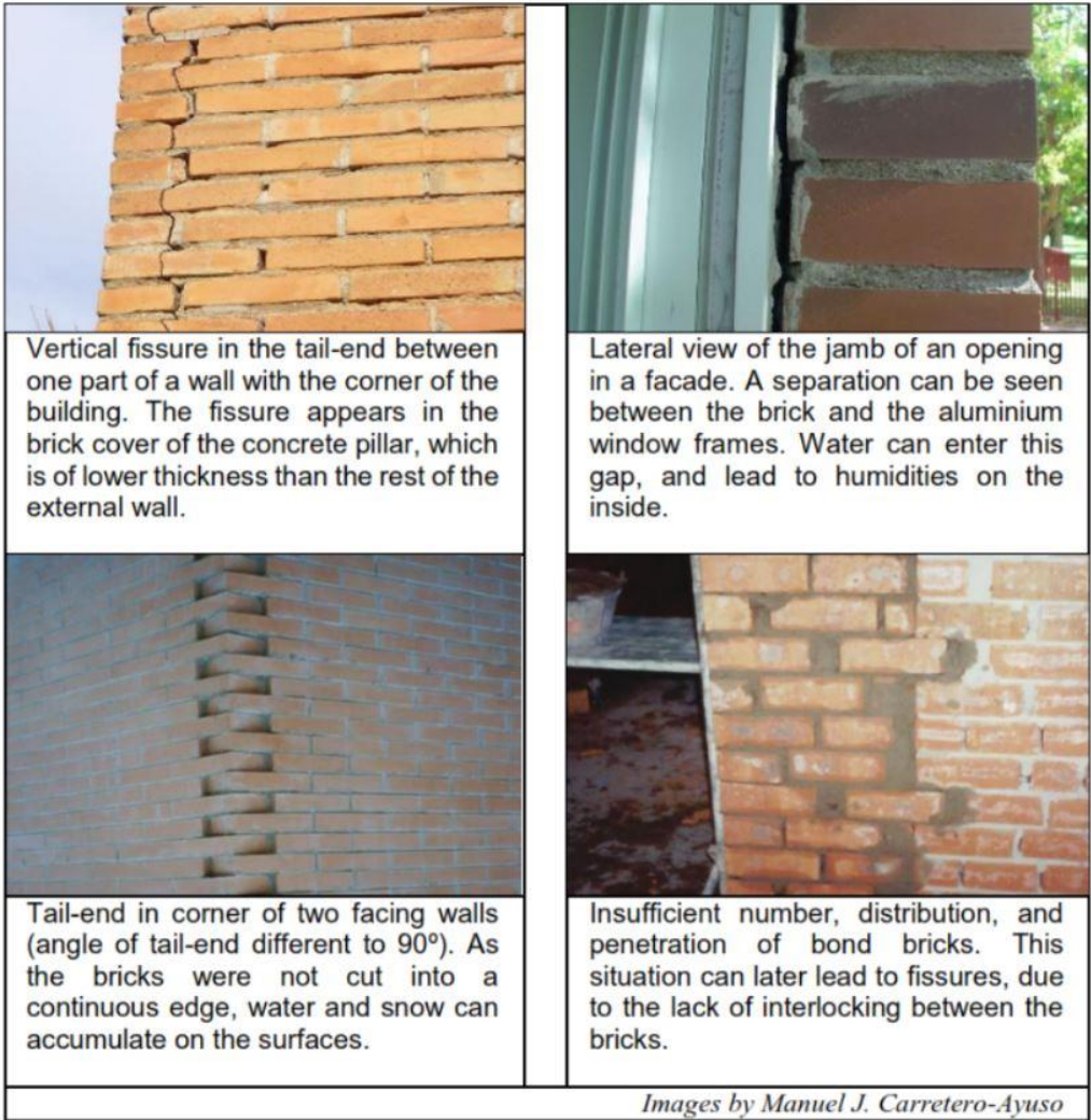
Figure 5 – Photographic examples of several execution problems
