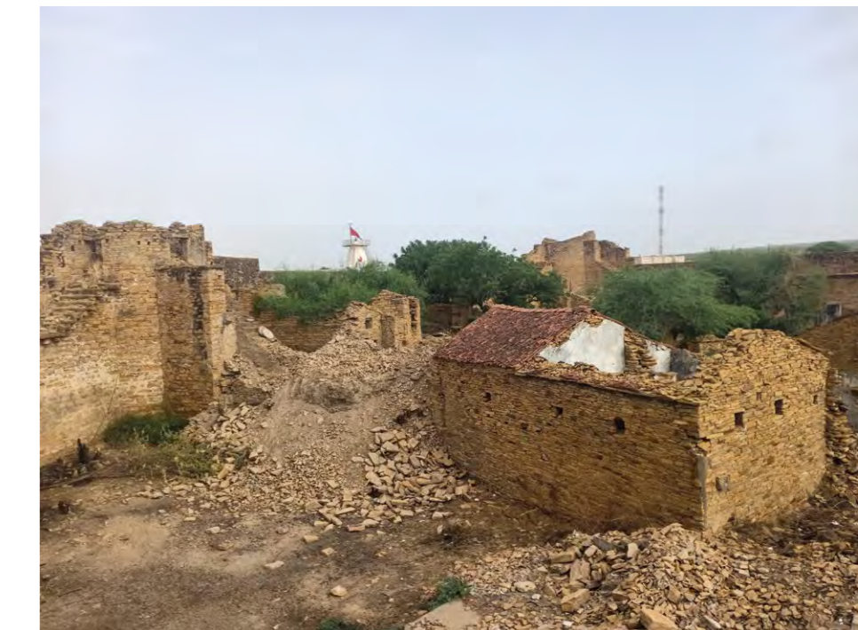
56. Photographic record of building 13 in Bela, with surrounding debris as marked in the previous figures. Photograph taken in the opposite direction of image 55, showing the back of the building.
