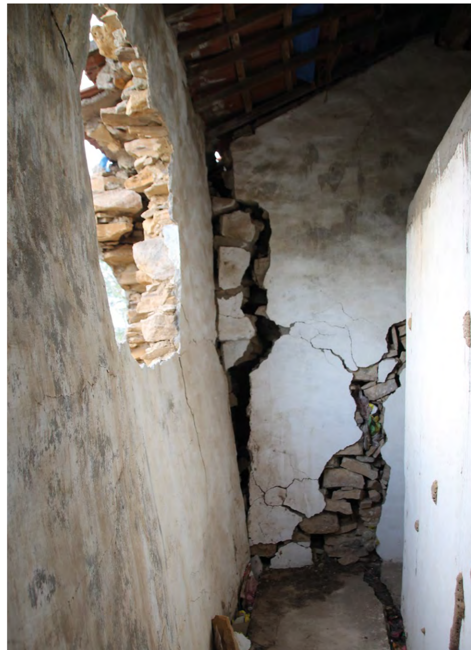
62. Internal view of Damage 2 (wall cracks) and portion of damage 1 (collapsed wall). Photographs can also serve as evidence of damage, but without accurate metric information as with 3DLS.
