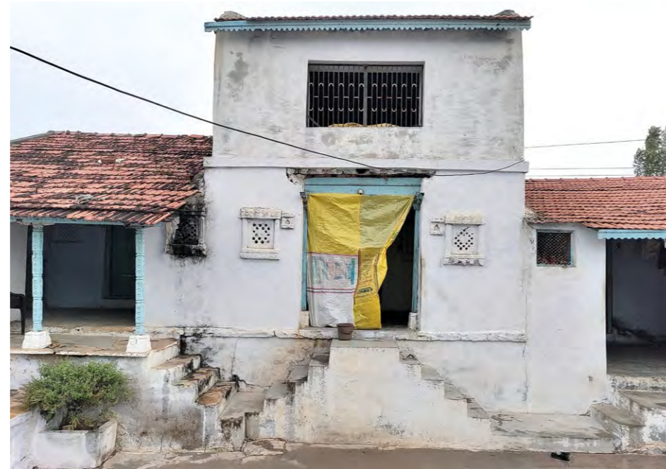
46. House 1 showing upper floor added to an existing single-storey building.
