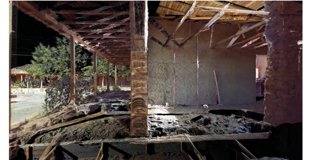
67. View of a dwelling affected by the 2010 earthquake in Lolol, Chile, with proposed storage-walls for materials and rubble to be re-used designed over the 3DLS data obtained on-site.
