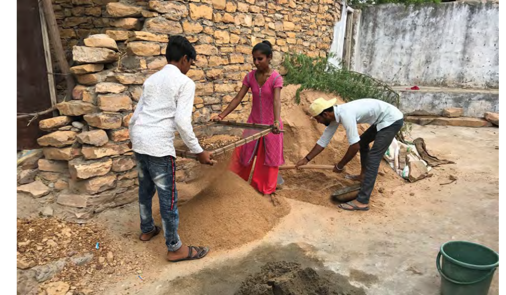
29. Community members building stone walls with cement mortar.
