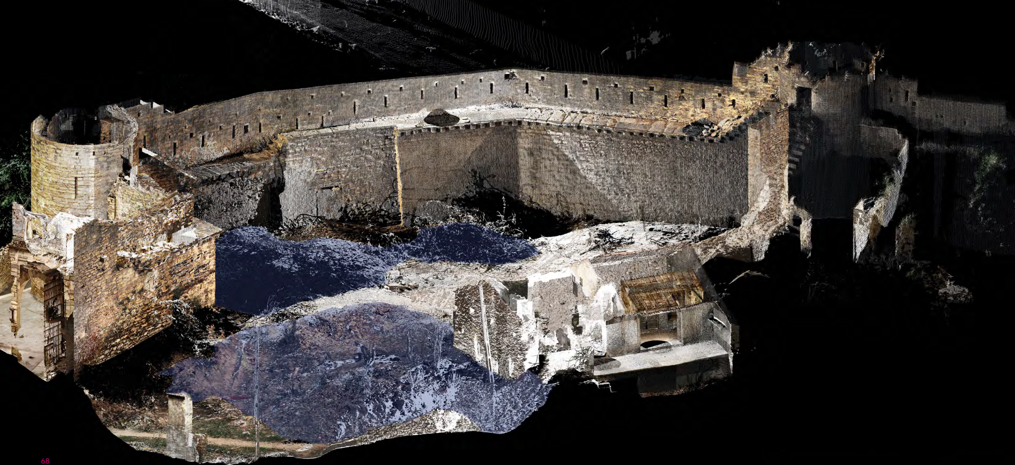
55. 3D view of building 13, with a partially collapsed roof and walls inside the Fortress in Bela. The surrounding rubble is marked in blue. The image was rendered from the 3D scanned data, using the same line profile as in section CC'.
