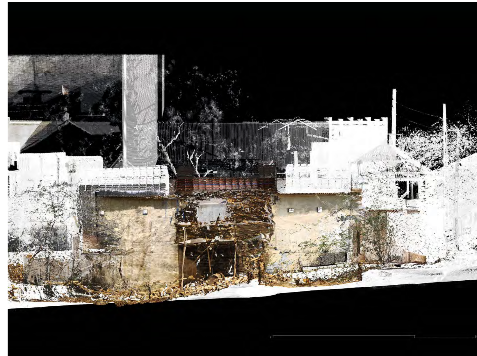
59. East elevation of temple 5 rendered from the 3DLS data in June 2021, showing the partially collapsed wall (damage 1).
