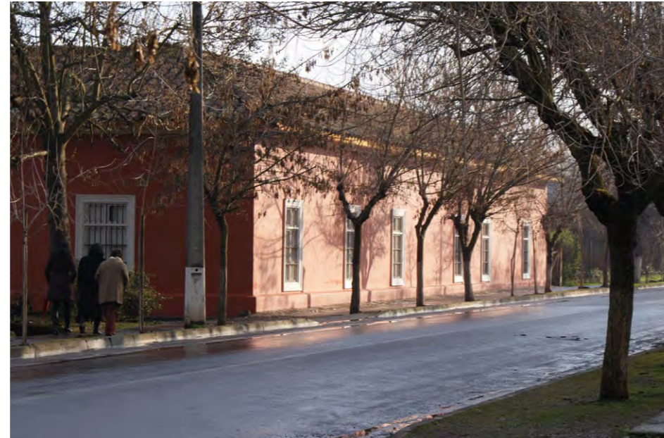
2. An adobe house with no damage after the 2010 earthquake in the historical village of Zúñiga, Chile, mainly due to regular maintenance and reinforcement.
