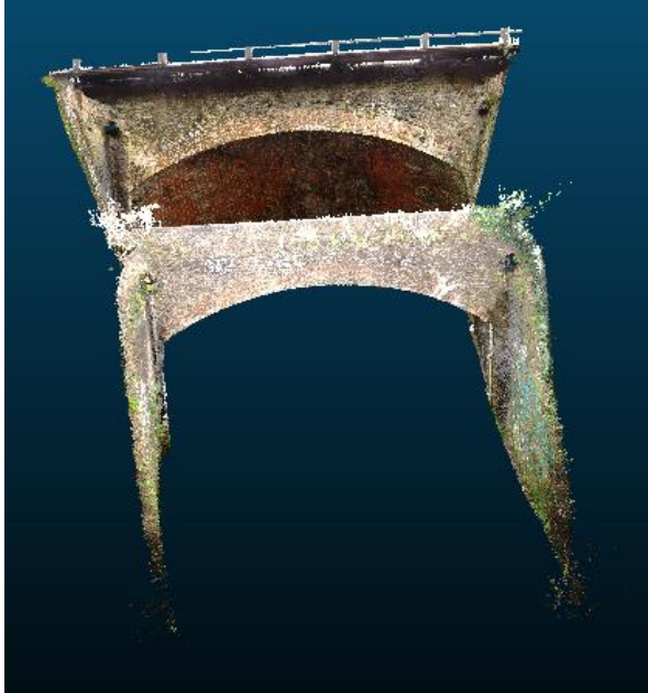
Figure 3. Cleaned and registered point cloud data of a masonry bridge.
