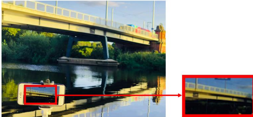
Figure 3-19: Camera focused on a portion of a structure
