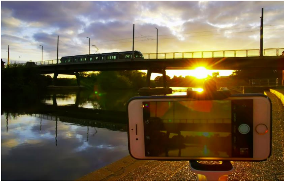
Figure 2-1: Nottingham Trent University (NTU)'s CV-based SHM set-up with camera focusing on a target section of the Wilford toll bridge in Nottingham
