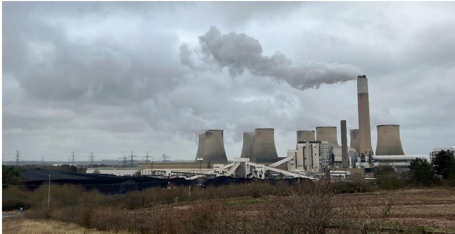
Image 2: Ratcliffe-on-Soar Power Station (11-01-2024)
