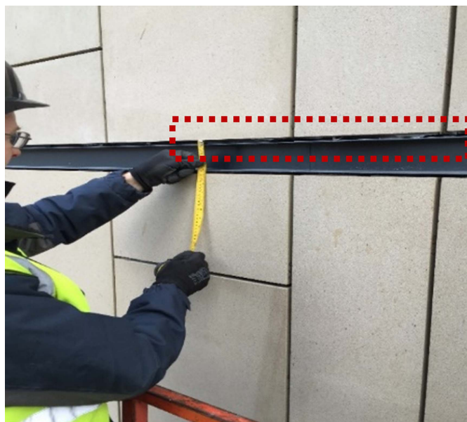
Fig. 5. Inconsistent gaps in some areas between the channel and the stone panel.
