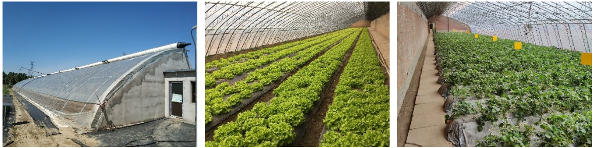
Figure 1.2 Outside (left) and inside (middle and right) views of the Chinese solar greenhouse. Soil culture is common in practical CSG production.
