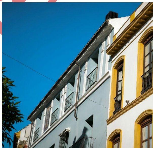
Figure 14. Detail of the upper floor of the house in 7 Cano y Cueto Street. September 2024.
