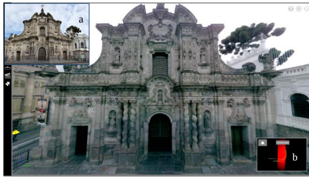
Fig. 1. a. Photograph of the main façade of the Church of the Company of Jesus in Quito; b. Leica Geosystems TruView TLS render.
