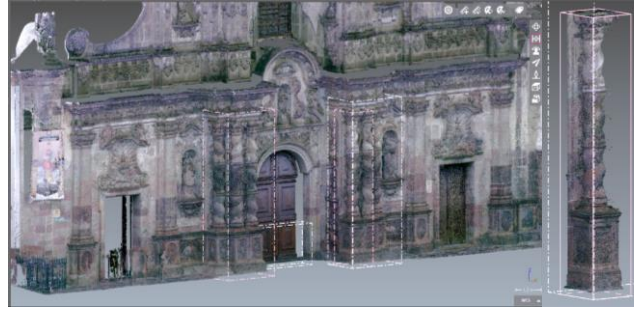
Fig. 3. Façade point cloud of the Church of the Company of Jesus with sectoring boxes for the Solomonian columns. Leica Cyclone 3DR software.
