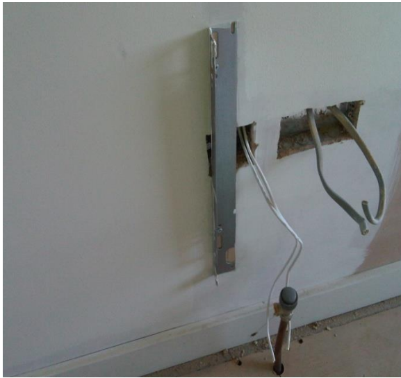
Figure 1: Hard clash on Site
